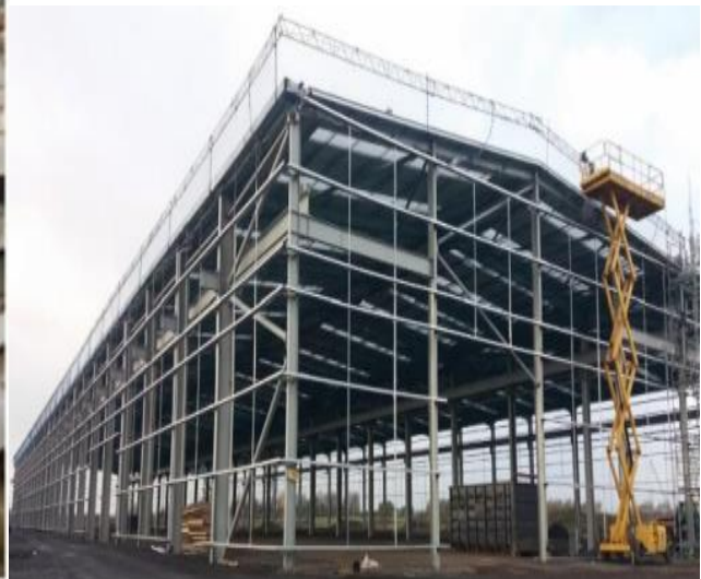
Fig.4. New Building with Reclaimed Steel
