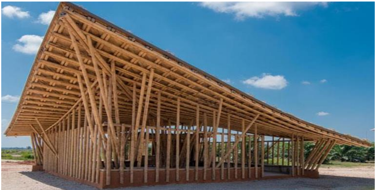
Fig. 2. Bamboo as a highly sustainable and versatile green building material
